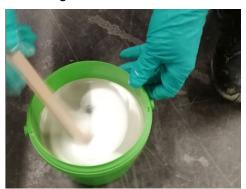
e) Application of liquid plastic "Wecryl R 230 Thix on both sides of the Zemseal® fully-bonded membrane according to the manufacturer's instructions with fleece insert.
