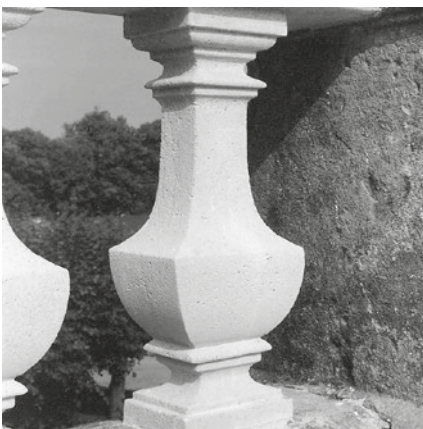
Perfect reproductions are achieved using white cement and sand followed by grit blasting.
