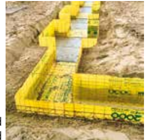
Pecafil® installed in-ground
