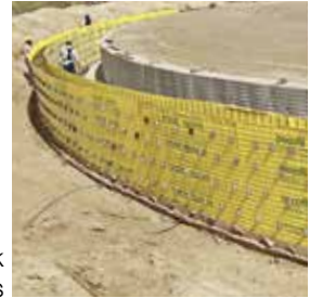
Circular formwork for foundations
