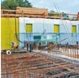
Pecafil® partition formwork, optionally with thermal insulation lining
