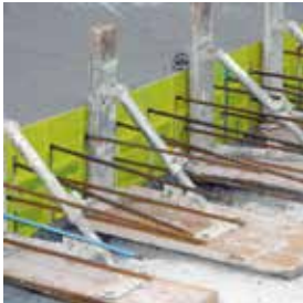
Formwork stop-end with continuity reinforcement
