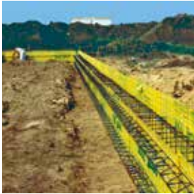
Installation of Pecafil® above ground
